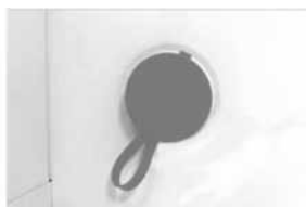
Fig. 5: Plastic plug for condensation drain (the plug seals the tank from the inside).
